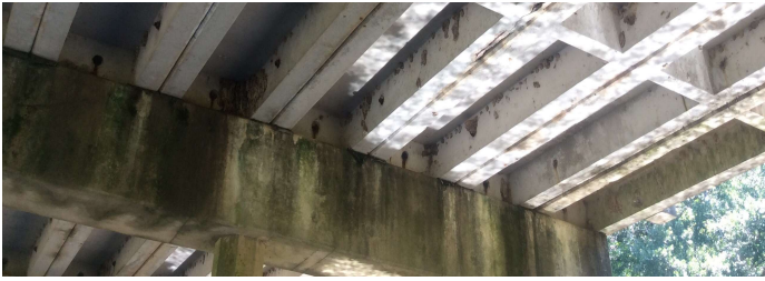
PHOTO 1 Description Span 5 Unit 5 left (delamination)
