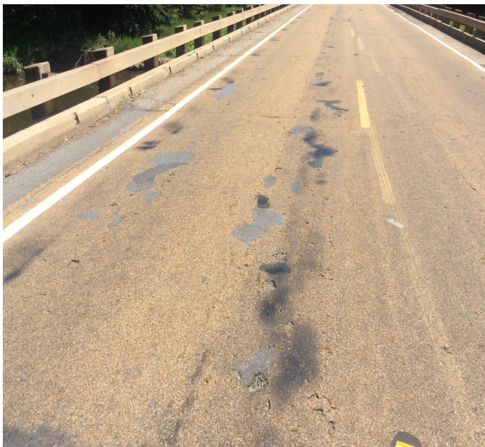
PHOTO 3 Description Wearing surface - Spans 1-2 (deterioration)
