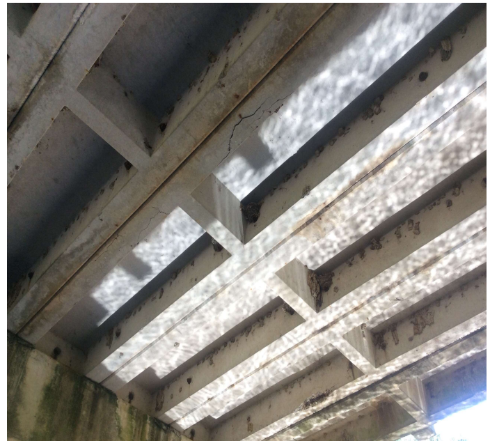
PHOTO 2 Description Span 6 Unit 7 right (rebar exposed)
