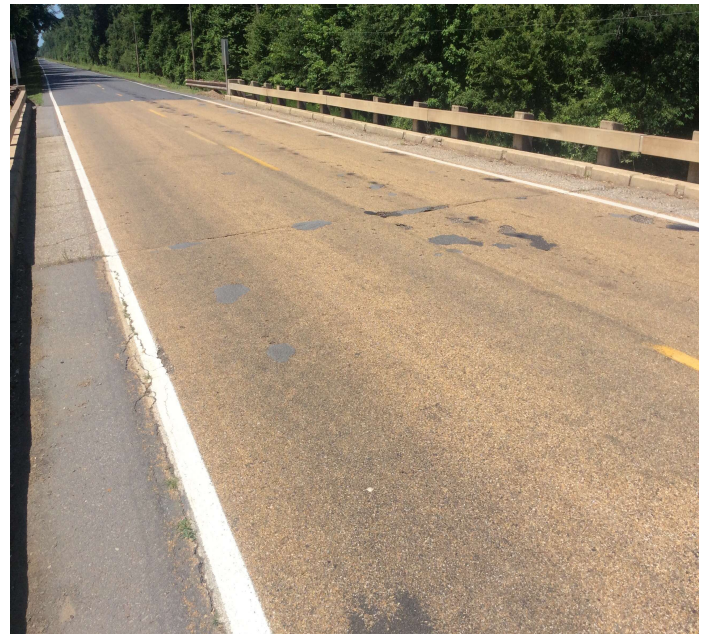
PHOTO 2 Description Wearing surface - Spans 3-4 (deterioration)
