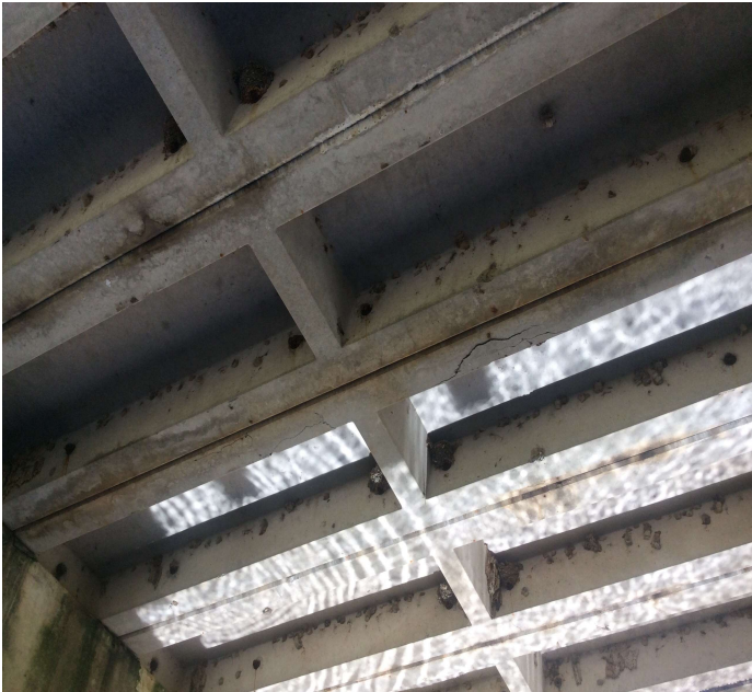
PHOTO 2 Description Span 6 Unit 5 left (delamination)
