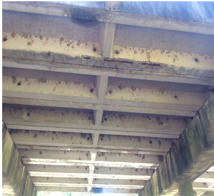
PHOTO 1 Description Span 3 Unit 1 right (rebar exposed)
