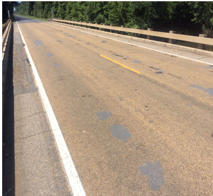
PHOTO 1 Description Wearing surface - Spans 6-8 (deterioration)
